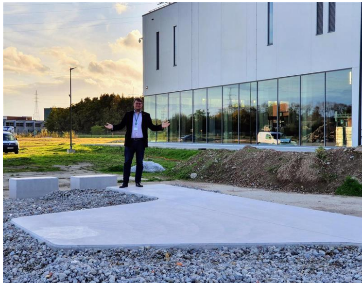
Bus stop/waiting area being constructed from mine tailings
